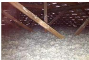
This home has a concrete tile roof. GreenWool handles moisture well, condensation will dry out and the wool will retain it's thermal efficiency
