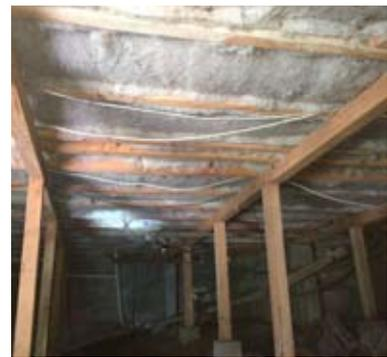
*Like the wall insulation, GreenWool Roll-Form Underfloor is stapled to the sides of floor joists to avoid sagging.*
